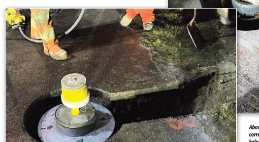
Above: Replacement of corroded light cans, used to help pilots navigate to and land at the airport.
